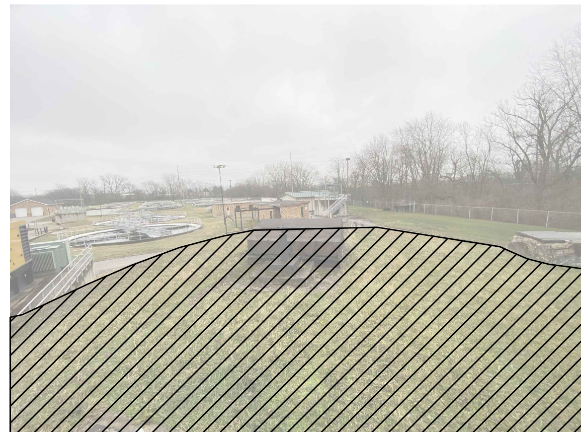
EXISTING BUILDING - ROOF
