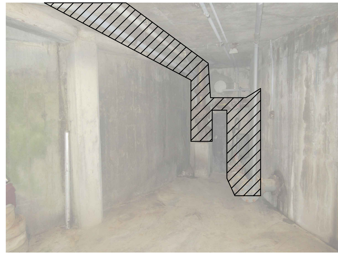
EXISTING BUILDING - BASEMENT
