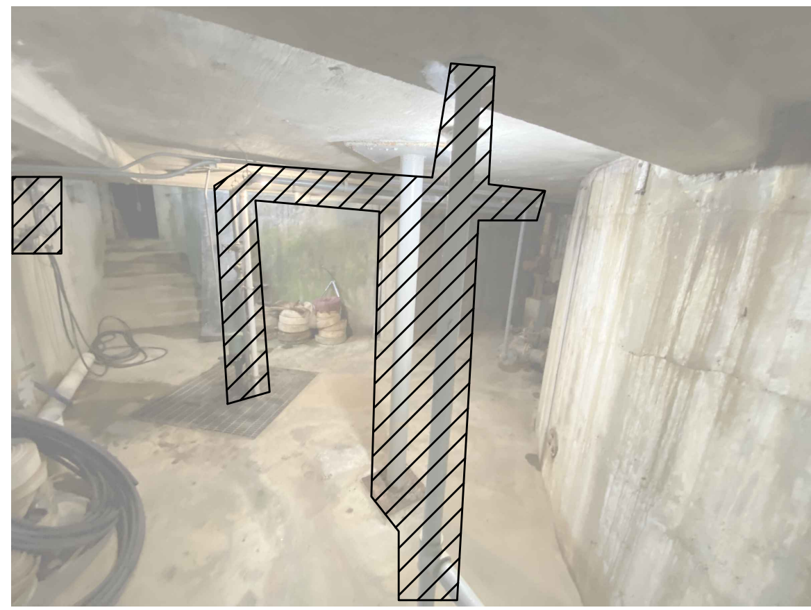
EXISTING BUILDING - BASEMENT
