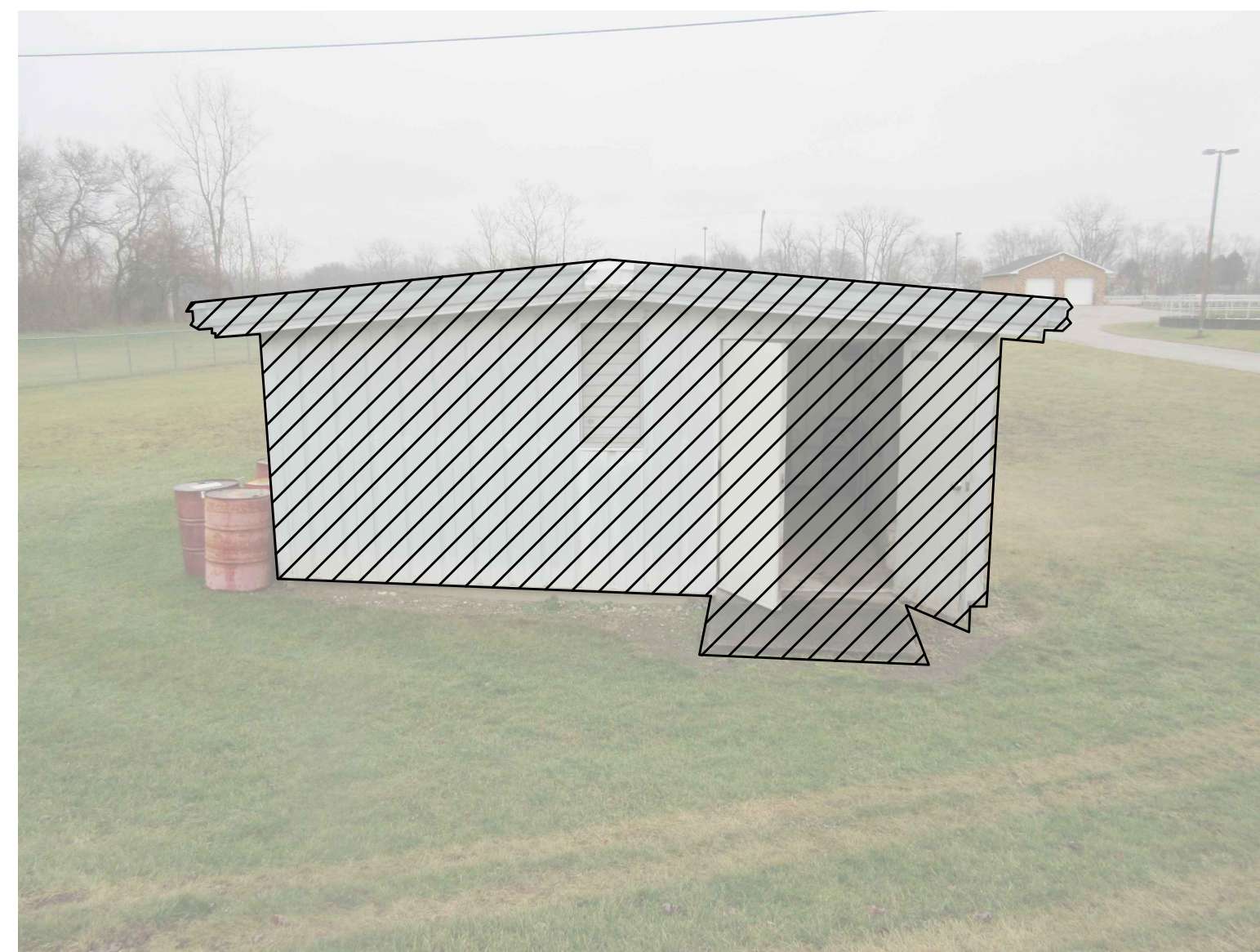
EXISTING STORM BASIN BLOWER BUILDING - WEST
