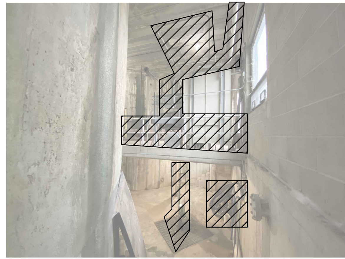
EXISTING BUILDING - BASEMENT
