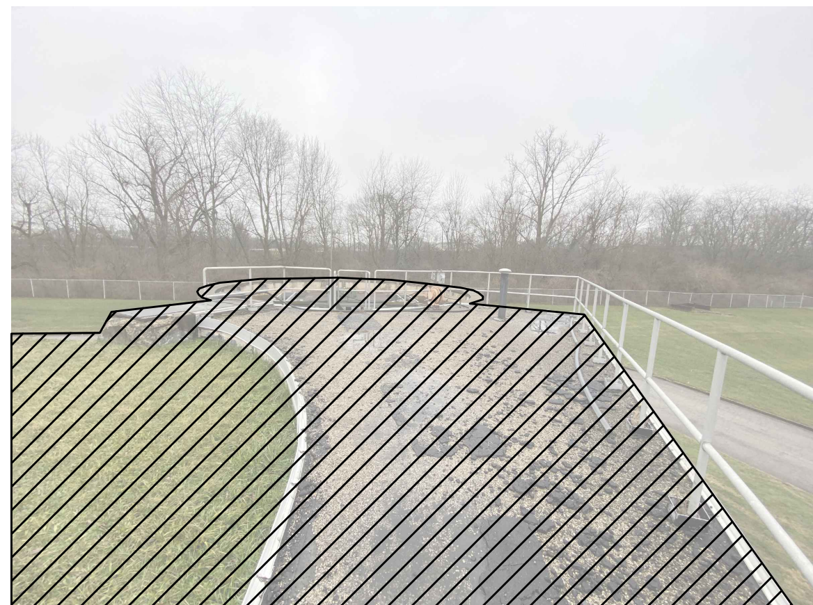
EXISTING BUILDING - ROOF
