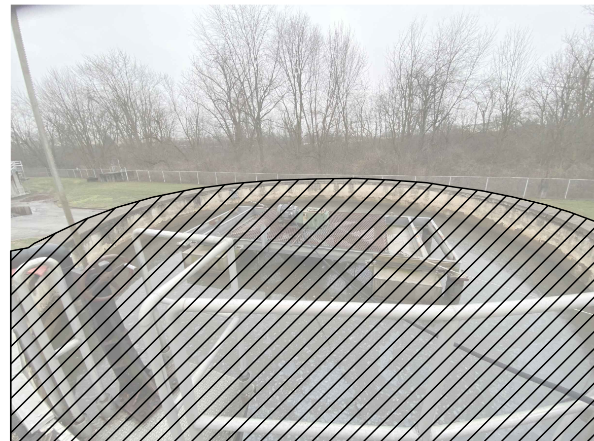
EXISTING SLUDGE HOLDING TANK - TOP
